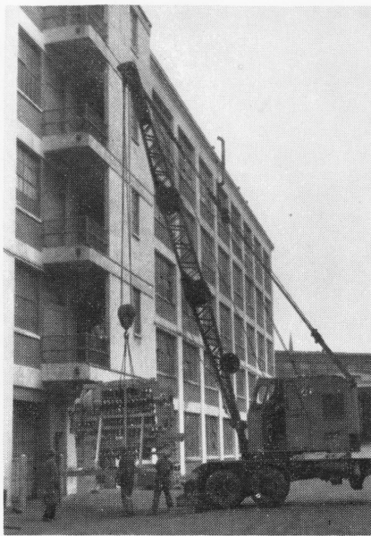
(Left) Angelo Poletta handles controls in the cab with which the giant eyelet machine will be lifted off the bed trailer. (Center) Foreman Charles Dubuque is on hand as millwrights Joe Milutis, Richard Duffy, Leo Ubaldi and Jerry
